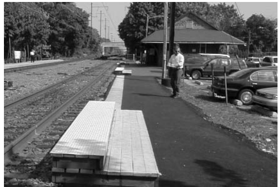
CCPC staff visually inspected each station to determine the condition, functionality and improvement recommendations.
