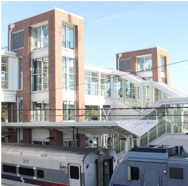
The new Paoli Intermodal Transportation Center brings the station into compliance with the provisions of the Americans with Disabilities Act (ADA) by including a new center high level platform, elevators, ramps, and a pedestrian overpass.
