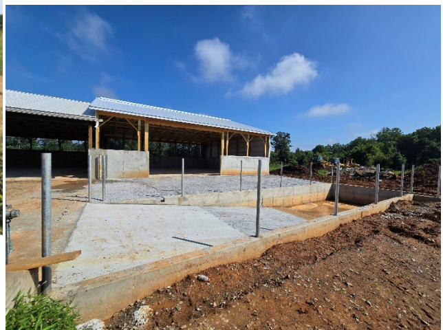
Figures 1&2: Southern Chester County beef cattle operation, before & after new roofed stack pad and heavy use area protection installation- Aug. 2025
